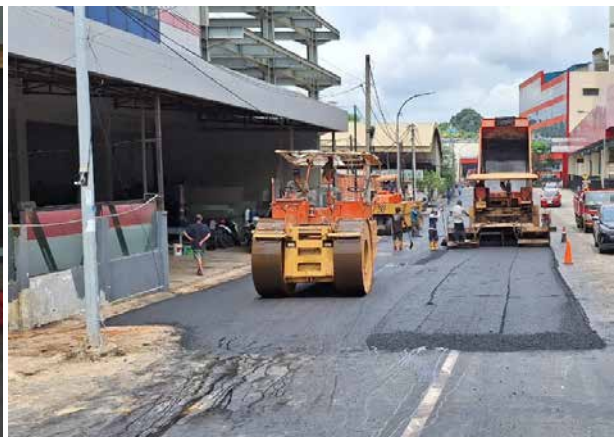
Road repair and re-paving activities
